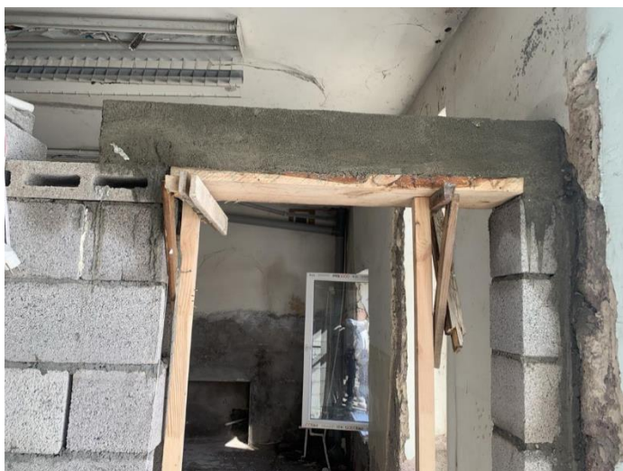
Reconstruction works are well in progress in Masis region, Ararat province. October 2023. © UNDP
